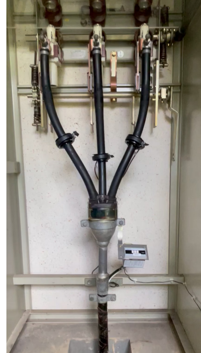
The type-tested design consisting of sensor and holder allows partial discharge-free operation for nominal voltages up to 11 kV.
